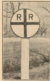
R. R. Crossing Sign (Circular) Standard in many states. Circular shape at railroad crossings only.
