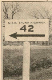
Night Sign (Rectangular) Placed at turns and set to catch automobile headlights. Especially useful for night driving.
