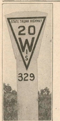
Mile Post Placed every mile. The number in the triangle is the number of the State Trunk Highway on which the mile post occurs. The number below the triangle is the Distance in Miles from the South or East Terminus of that State Trunk Highway.
