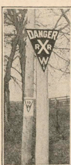
Danger Sign Placed for your protection at places where there is real danger: R, R, grade crossing, sharp turns and abrupt hills. Center lettering indicates reason for the warning.
