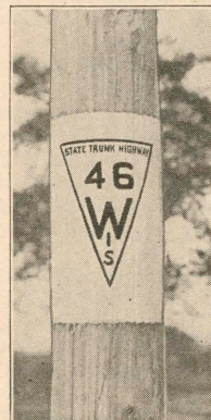
Direction Sign Placed at intersections on the State Trunk Highway System to guide the traveling public. The best roads to places off the System are indicated by signs of like general character set at the proper intersections. The figures indicate distances in miles.
